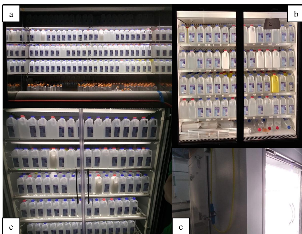
Figure 1. Retail display cases for milk bottles. a: display case 1, open-shelf, 10820 lux; b: display case 2, glass-doored, 670 lux; c: display case 3, walk-in, 3790 lux.
